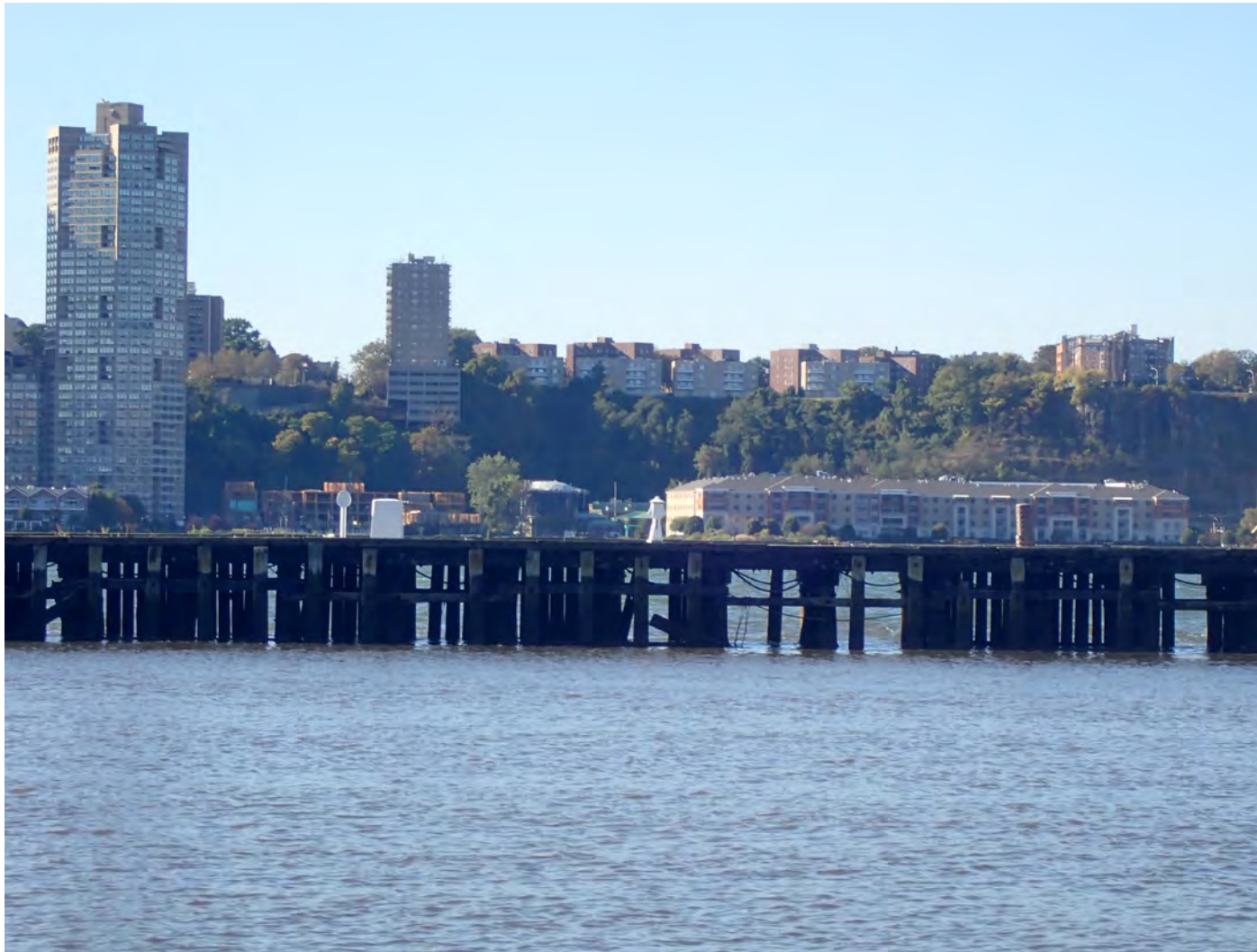
1 - View Looking West at Wave Screen
