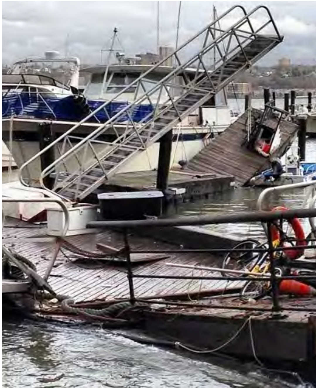
Dock & Gangway Damage
