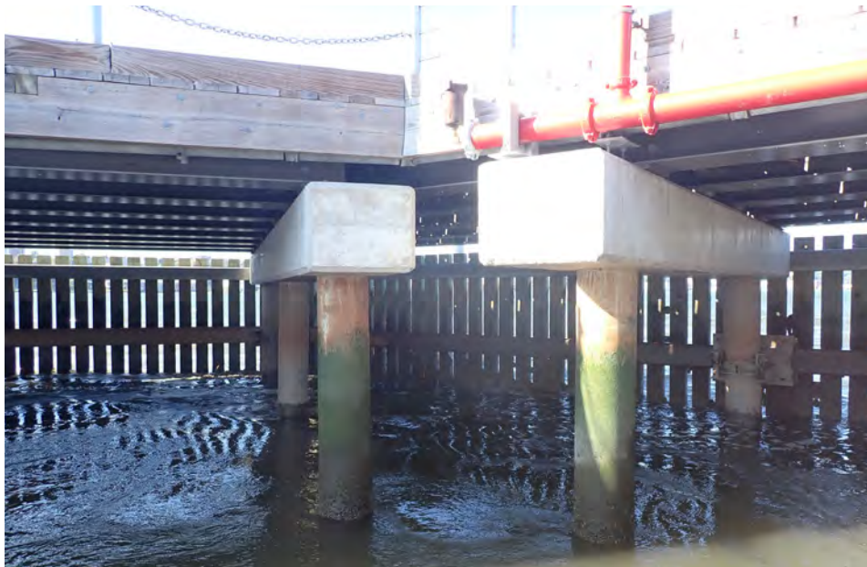
Steel Piles & Concrete Pile Caps
