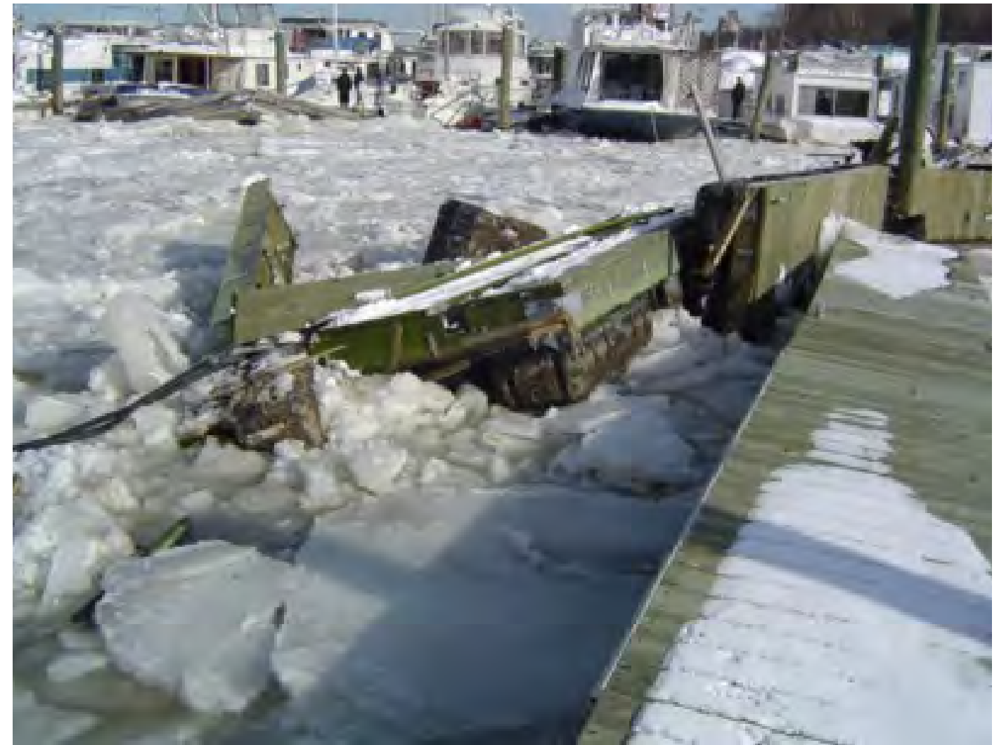
View from E-Dock Looking North at D-Dock Ice Damage
